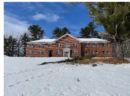
Existing vacant building on EYDC campus
